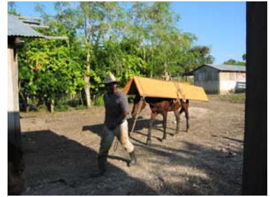
They bring boards in two at a time to construct a church building.
